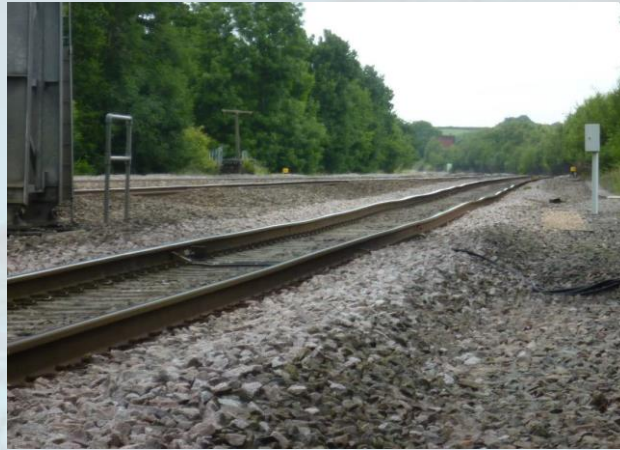
Figure 2. Intense deterioration of track geometry as a result of low track stiffness
